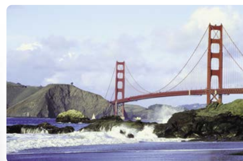
Golden Gate Bridge
