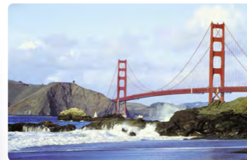
Golden Gate Bridge
