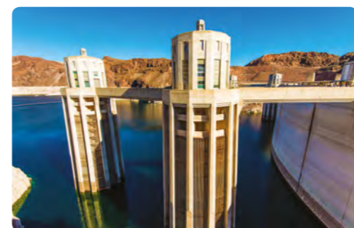
Hoover Dam intake towers
